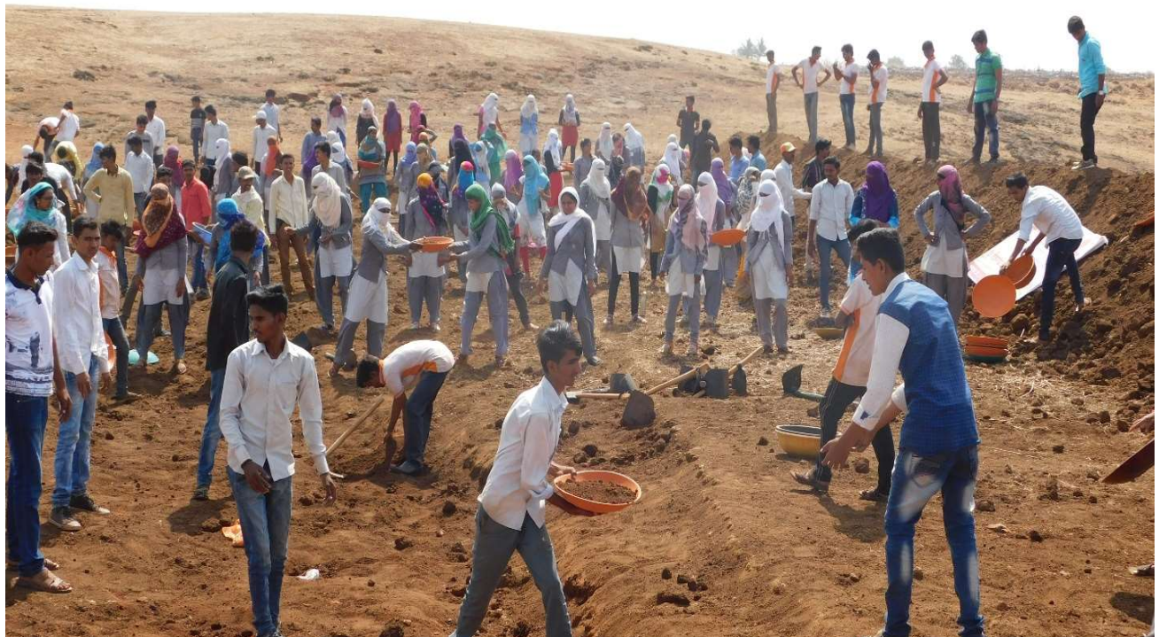
Mati Bandhara (Soil Dam) - water storage capacity - 1000 QM
