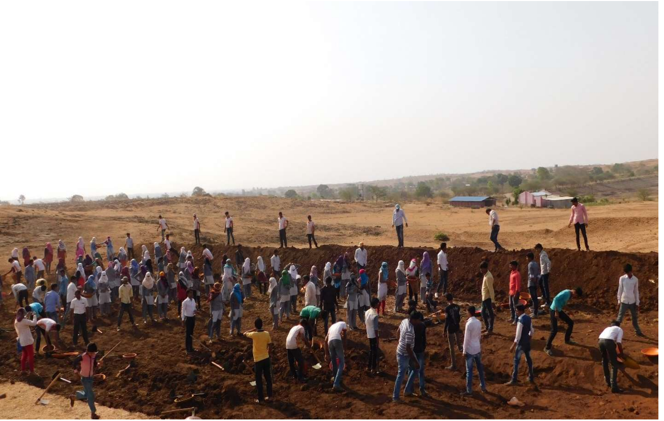
Mati Bandhara (Soil Dam) - water storage capacity - 1000 QM
