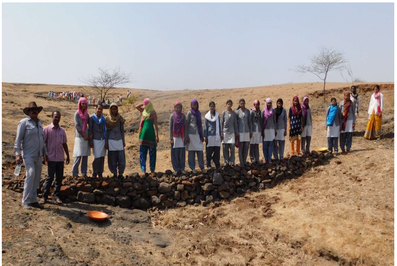
Volunteers constructed 30 Small Stone Dam (Dagdi Bandh)
