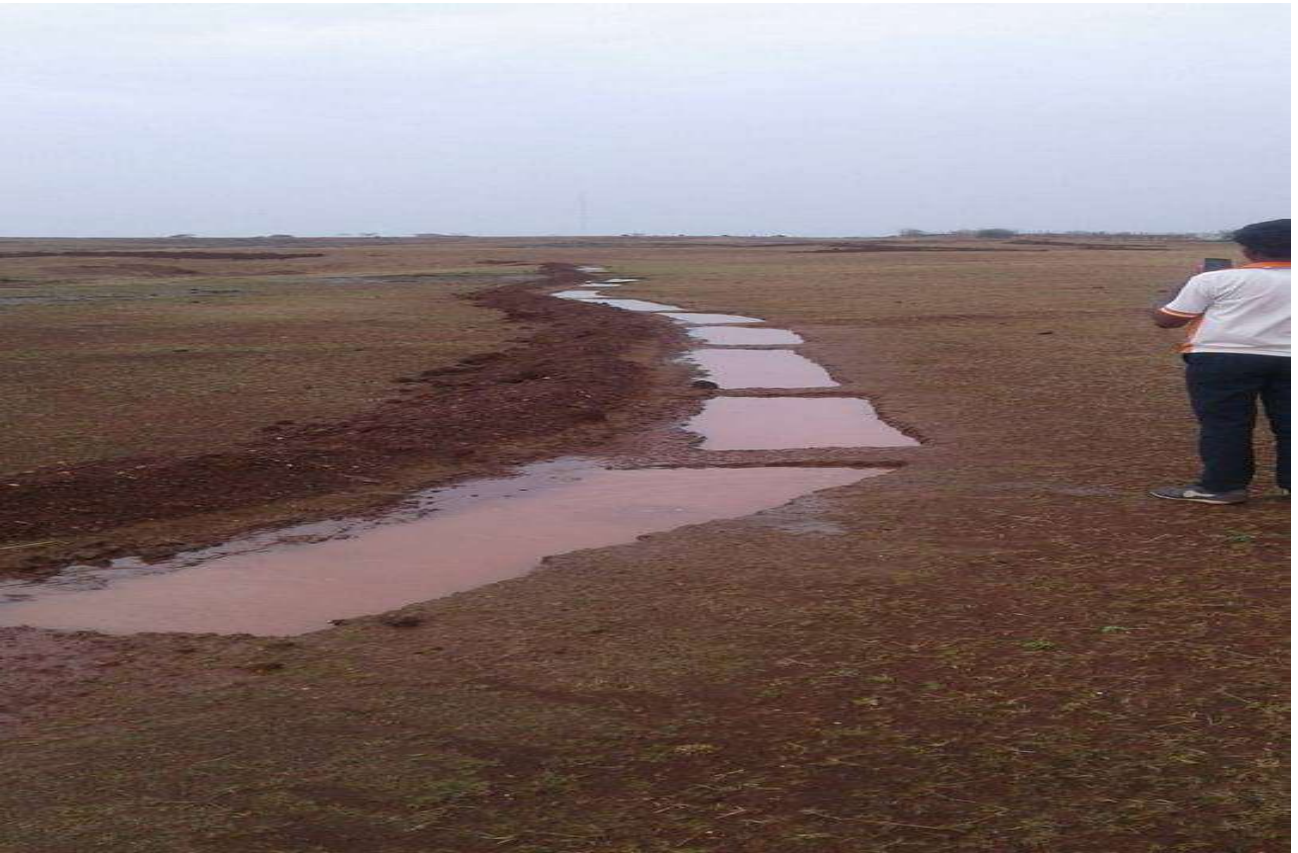
Water in CCT's after Rain - 20/06/2018
