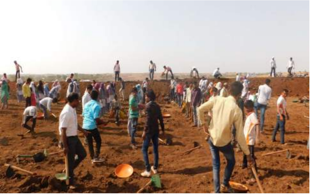
2 nd Mati Bandhara (Soil Dam) - water storage capacity - 1500 QM
