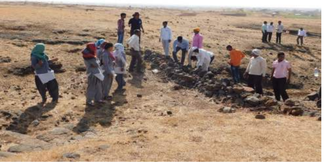
Some Villagers were also participated in constructing a Small Stone Dam (Dagdi Bandh).
