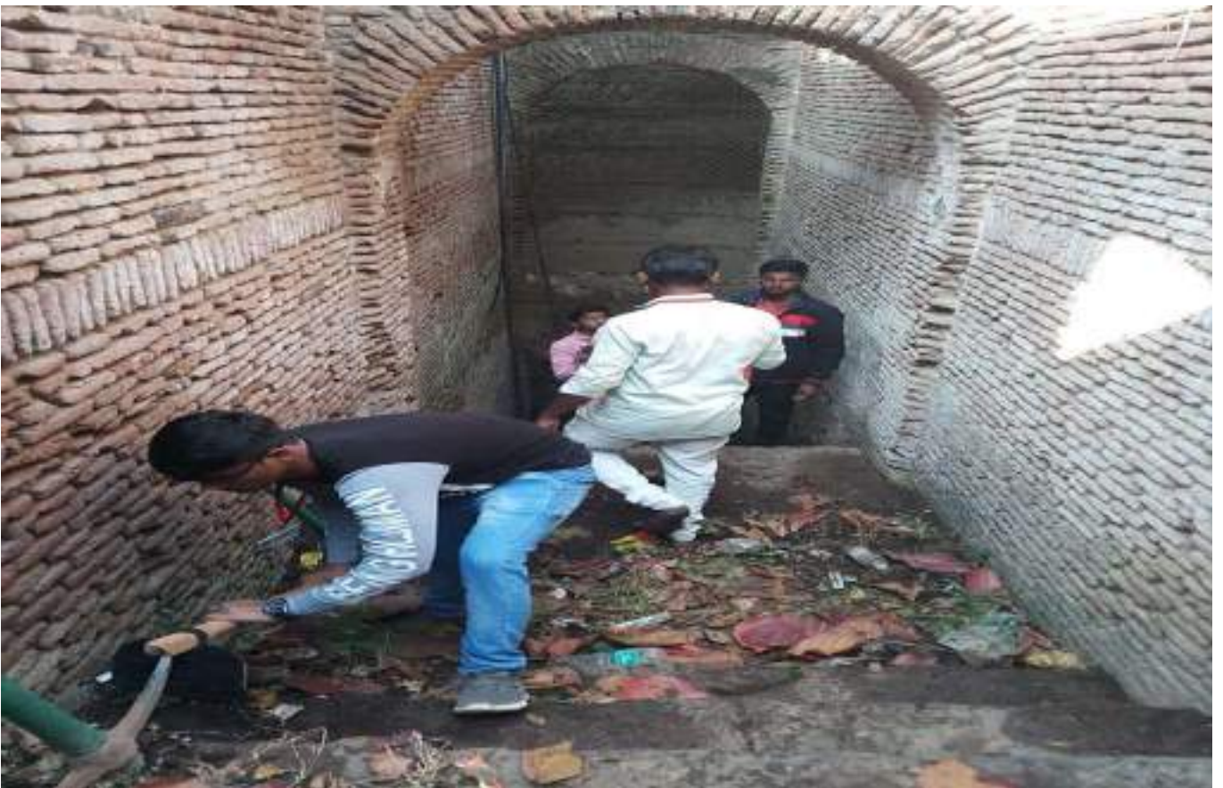
Cleaning of old water Source (Ahilyabai Barav) at Dhongavhan Wadi.
