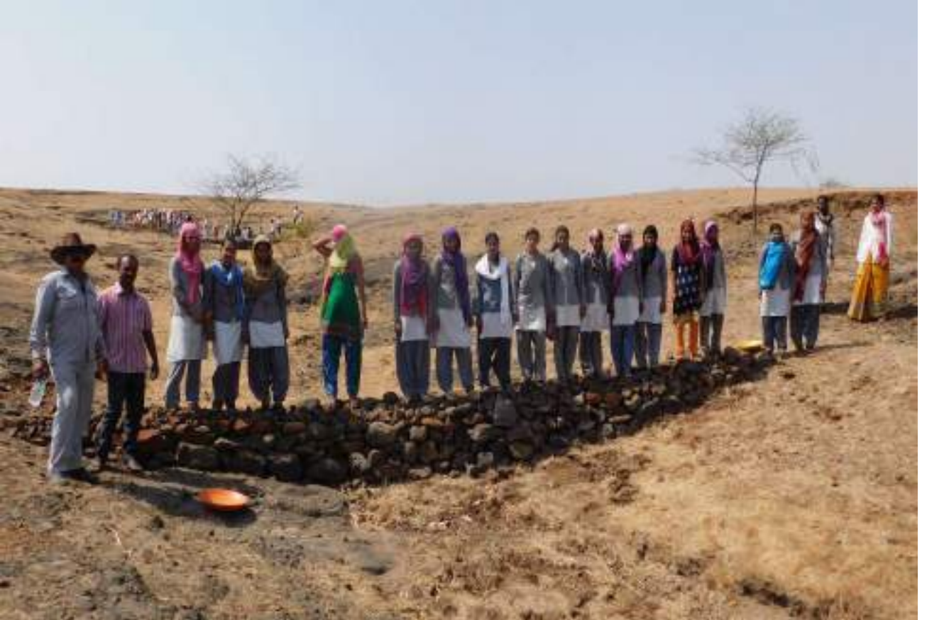
Volunteers constructed 30 Small Stone Dam (Dagdi Bandh)
