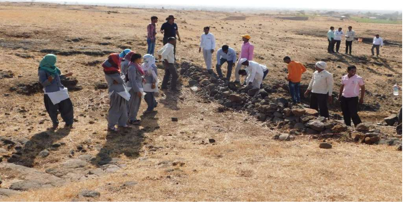
Some Villagers were also participated in constructing a Small Stone Dam (Dagdi Bandh).
